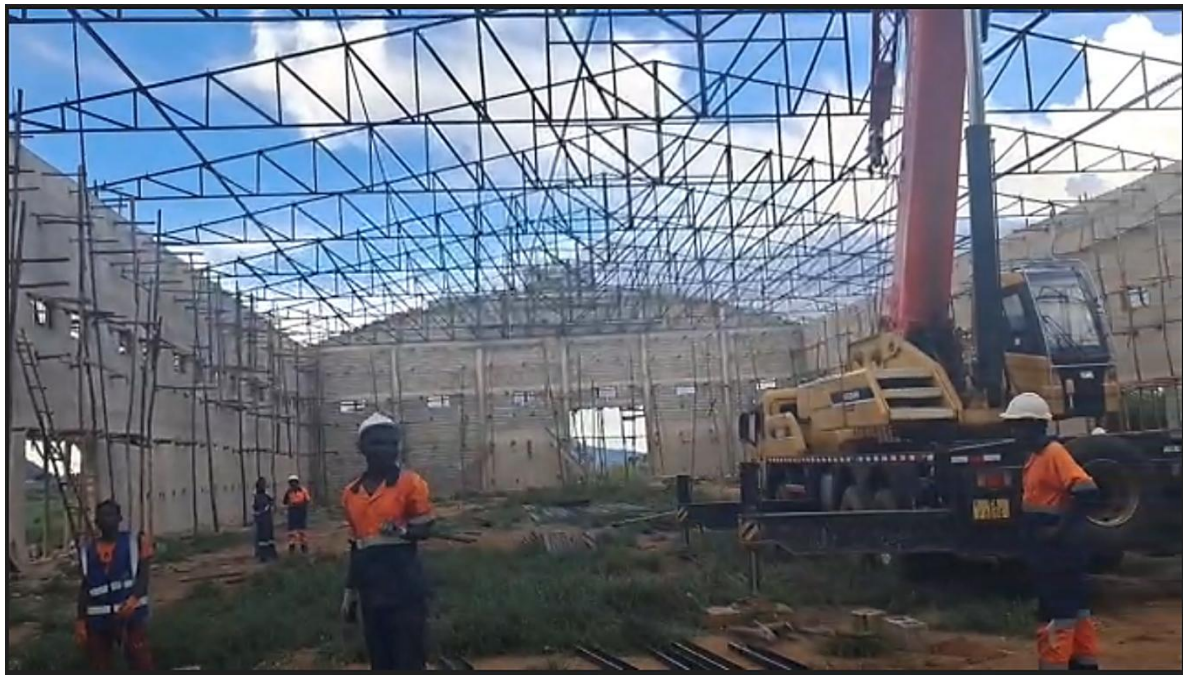
Photo: Speedy’s new warehouse under construction. Credit: Growth Poles Project
